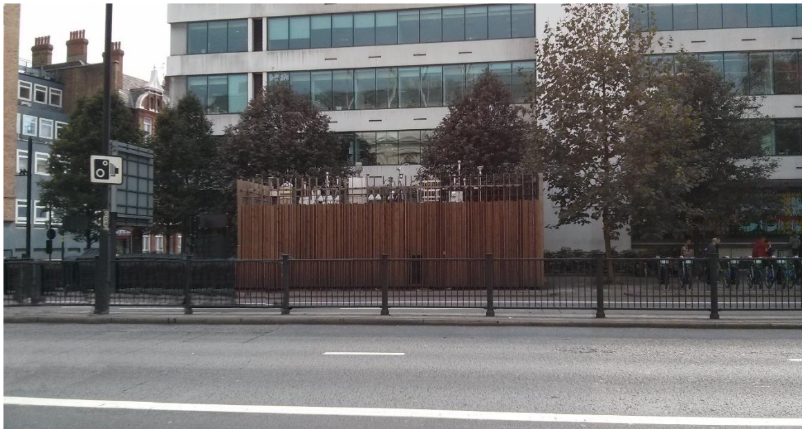
Figure 1: Front side of monitoring station along Marylebone Road.
